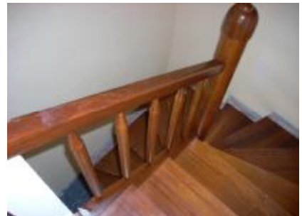
Staircase to the first floor
